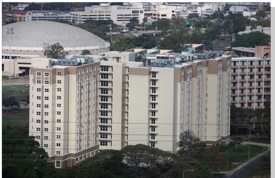
The size and number of rooms in the University of Hawaii at Manoa's Frear Hall presented plenty of hurdles, but Daikin cleared them all so easily the building is now LEED ™ Silver certified.
