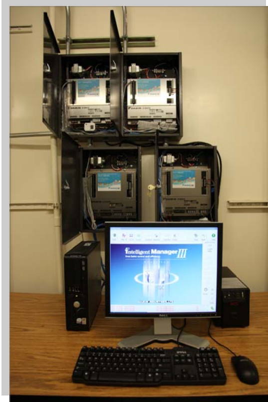
The Intelligent Manager III gives the staff the ability to restrict, turn off or setback individual dorm room air conditioners from their offices prior to leasing and occupancy.
